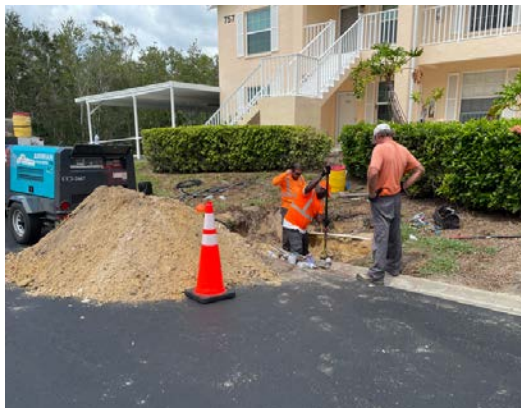
The connection to potable water is being completed by Collier County workers.
